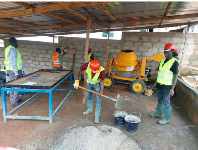
Photo: batching and mixing of concrete
