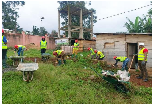
Photo: clearing and cleaning of the production site
