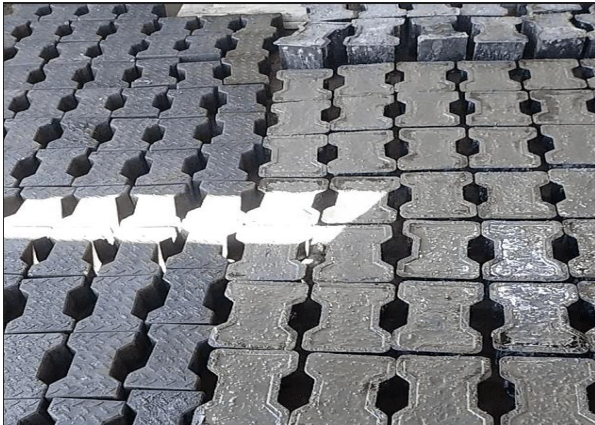
Photo: demolding of pavement blocks
