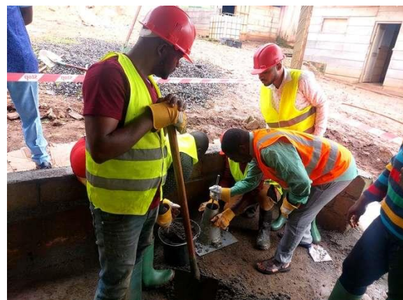
Photo: geotechnician carrying out concrete slump test
